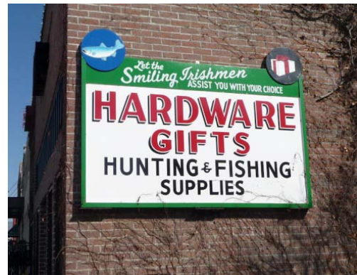
Figure 8. Acceptable firewall sign example.
