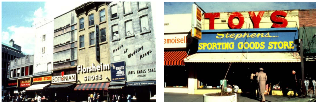
Figure 7. Unacceptable wall sign examples. These signs are out of scale with the facades and appear to cover over historical architectural features.
