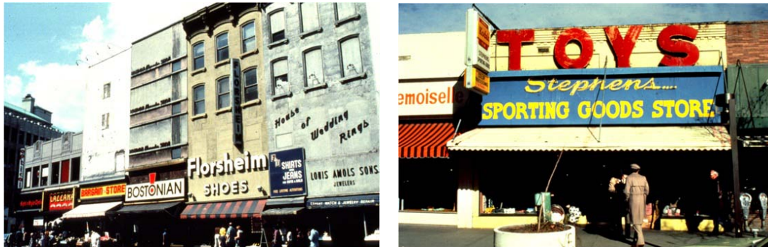
Figure 7. Unacceptable wall sign examples. These signs are out of scale with the facades and appear to cover over historical architectural features.
